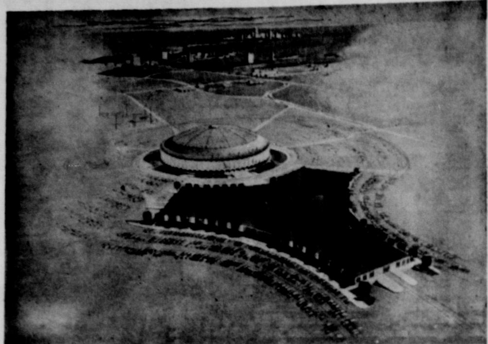
HOME OF HOUSTON LIVESTOCK SHOW AND RODEO —The largest livestock exhibition building under one roof in the world will be the home of the Houston Livestock Show beginning in 1966. The air-conditioned building covers 12 acres and will have stalls to accommodate 1700 halter cattle, 600 horses, 1200 swine, 1200 sheep and goats, and a 208 x 80 livestock judging arena. It will provide separate sheep and swine arenas, an auction arena for breed sales and commercial cattle, facilities for poultry and rabbits and a milking parlor with observation facilities. The exhibition building is adjacent to the famed Domed Stadium which will house America's largest and wildest rodeo.
