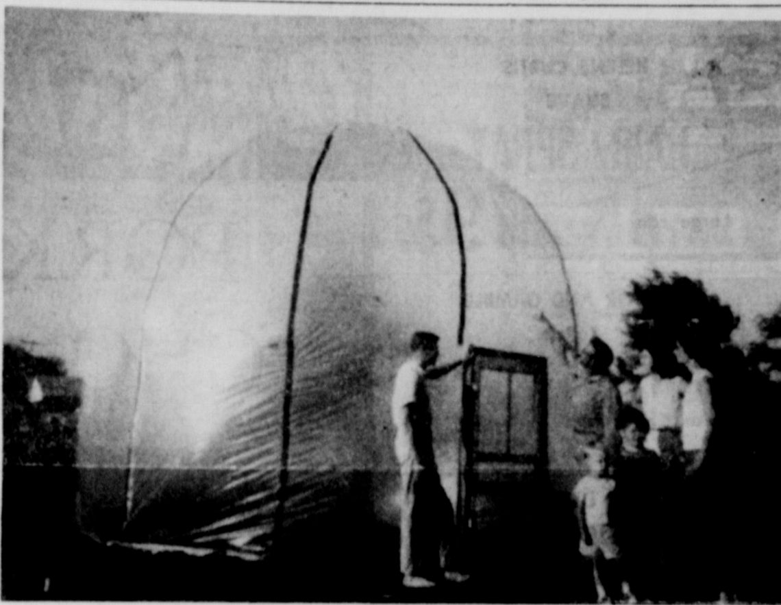
BLOWN UP: Builders of the new plastic hot house step back to admire their work. From left, the adults are Perry Isom, Petite Everett, Mrs. Everett and Mrs. Isom. The little ones are Gregg Isom (left) and Perry Everett. The plastic igloo keeps its shape through the use of a small blower. (McLean News Photo)
