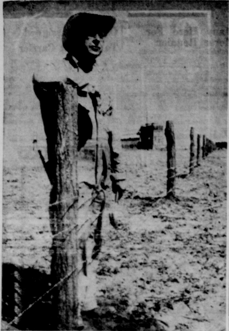
CROSS FENCE: Harris King is standing by a fence he is constructing on his farm northeast of McLean. Purpose of the fence is to protect an area seeded to grass this year and for better distribution of grazing. King also has done 55 acres of range seeding and constructed another fence. He did this work through the Great Plains Conservation Program.
