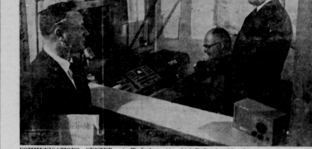
COMMUNICATIONS CENTER at Wadesboro, N. C., combines a round-the-clock civil defense nerve center with a unified radio service for local police, fire and sheriff's departments. Used for this dual purpose, the equipment is kept in top notch condition at all times to meet emergencies. At the radio is Waldo J. Stroud, one of three op- erators hired by the local CD unit under a program in which Federal and local governments share the costs of new civil defense employees. Raymond H. Northcutt (right), Wadesboro-Anson County CD director, explains his radio setup to Herman J. Sisk, Area E director for the North Carolina Civil Defense Agency and one of five area directors hired under the same cost-sharing law to help build up CD at the local level. (OCDM Photo)
