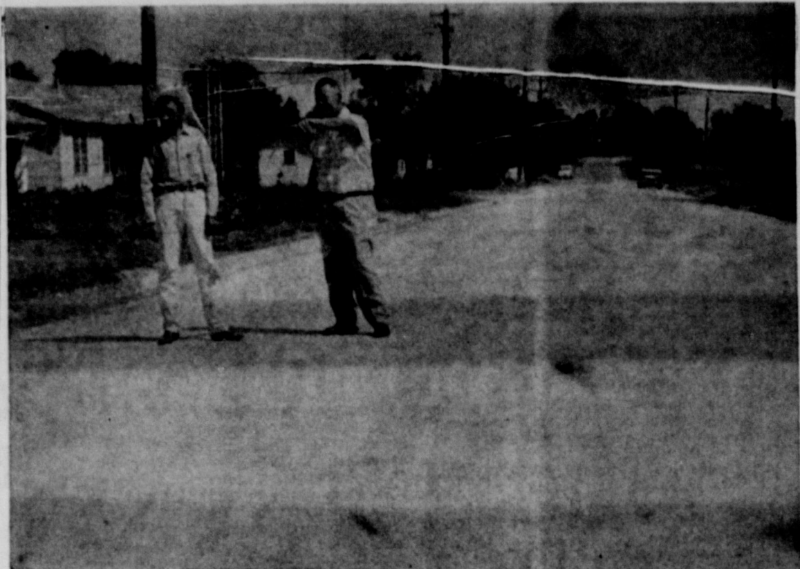
NEW STREET: City Manager B. J. McCartney (right) shows Mayor John Haynes one of the new blocks of streets constructed this year by city employees. This block, between Seventh and Eighth on Main, was one of 8 1/2 completed during the spring and summer. Repairs were made to several other streets, and a seal coat was poured on 17 older blocks. (Staff Photo)
