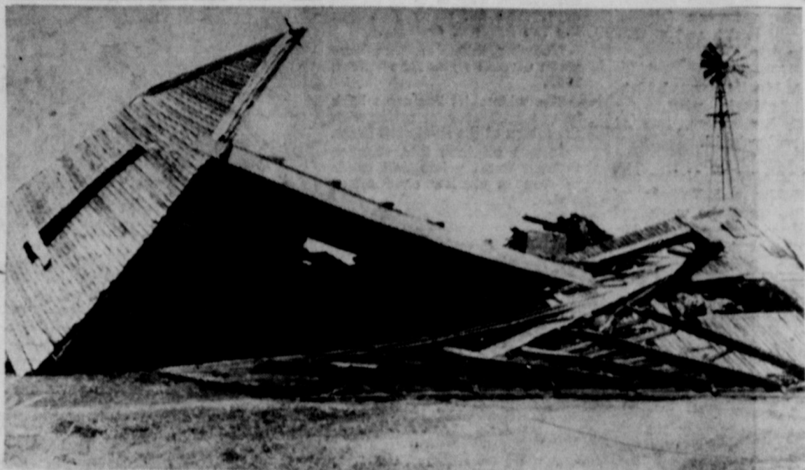
IN WAKE OF TWISTER —Shown above is the shattered structure three miles north of McLean on the Lefors highway that was hit Sunday afternoon by a twister during the violent storm that crossed the McLean area. The small tornado went on to break five telephone poles and damage nearby homes before it subsided.
