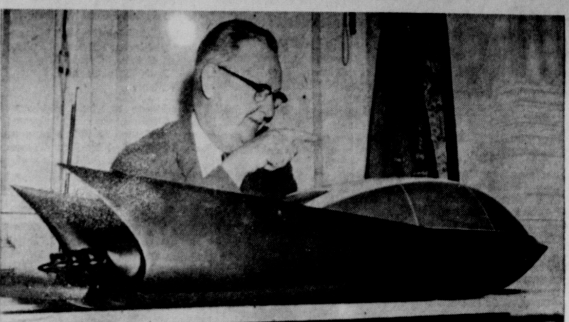
AIRBORNE GROUND VEHICLE —"Levacar" is the name of the strange-looking device being examined by House space committee chairman, Rep. Overton Brooks (D-La.), in Washington. One of several vehicles-of-the-future shown in model form to the space committee members, it rides on a thin cushion of air instead of conventional wheels. Predicted top speed: 500 m.p.h. Hose attached to vehicle at extreme left supplies compressed air to the working model. Self-contained blowers would do the job in the actual machine.
