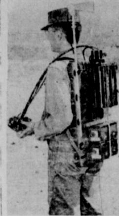
WALKING RADAR — New, lightweight version of radar can be back-packed by a soldier, as demonstrated at Fort Huachuca, Ariz., by the Signal Corps.
