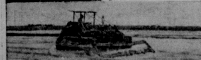
SEA OF MUD —An unusual sight near Agua Dulce, Tex., is this International TD-14A crawler tractor, spreading a "sea of mud," which results from salt water pits. After the tractor, equipped with the special mud-spreader, has done its leveling job, the mud dries and the earth is returned to its original condition.
