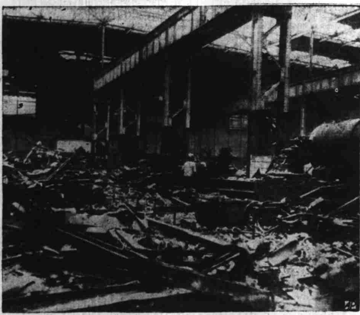
DESTRUCTION OF MACHINERY OF WAR —Steel girders and rubble strew the floor of one of the buildings of the huge Krupp works at Essen, Germany, which is being dismantled. Sections of the great steel plant used in making armaments are being destroyed. (AP Wirephoto.)
