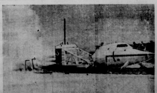
PRELUDE TO SPACE—The forebody of the X-15 research rocket plane roars down the of the Experimental High Speed Track at the Hight Test Center, Edwards Air Force Base, The sted run is one of a series designed to test the performance of the pilot's suit, what the fitted on a dummy inside the cabin. Information gathered will give some of the answer
