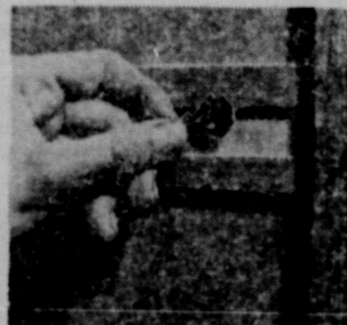
Insert patented clip in groove of each furring strip.
