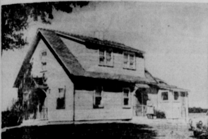
The new-looking home above is an example of imaginative remodeling. The "before" version is shown at the left. After structural changes, including a new foundation, new blended green asphalt roof shingles and new siding, pastel green in color, were applied. Wood windows were painted white to complete the exterior decoration of the house.
