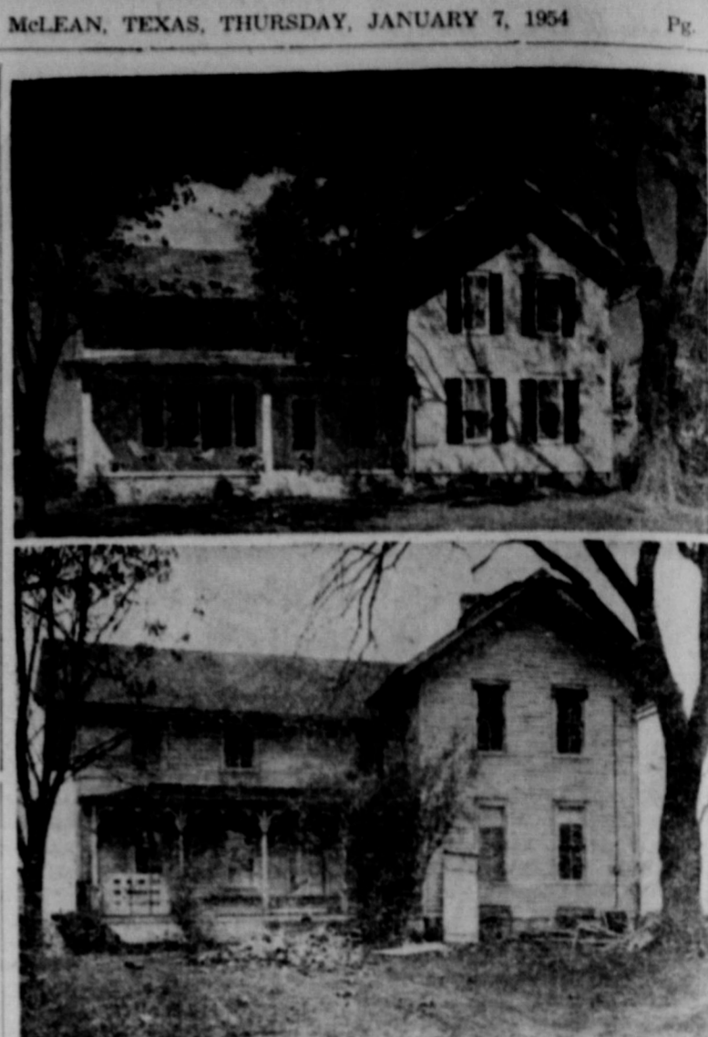
Remodeling gave clean, modern lines to the old house shown above in "before" and "after" versions. A new roof of colorful asphalt shingles, new paint for the sidewalls, and shutters were major changes.
