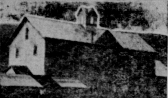
A remodeled barn is shown at the right side of the group of buildings above. The barn before modernization is at the right. Re-roofing with colorful asphalt shingles, new paint and new windows were main exterior improvements.
