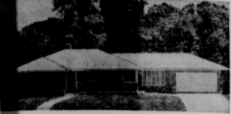
Silver-gray asphalt roof shingles are typical of the modern look in building materials. Light-colored roofing draws the eye upward making a low house seem taller than it actually is.
