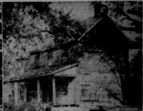
now protect this historic dwelling from weather and fire. The dark roof also offers pleasant contrast with the white asbestos-cement siding, and it helps to make the house look lower than it actually is. A light or bright roof would make the house seem higher.
