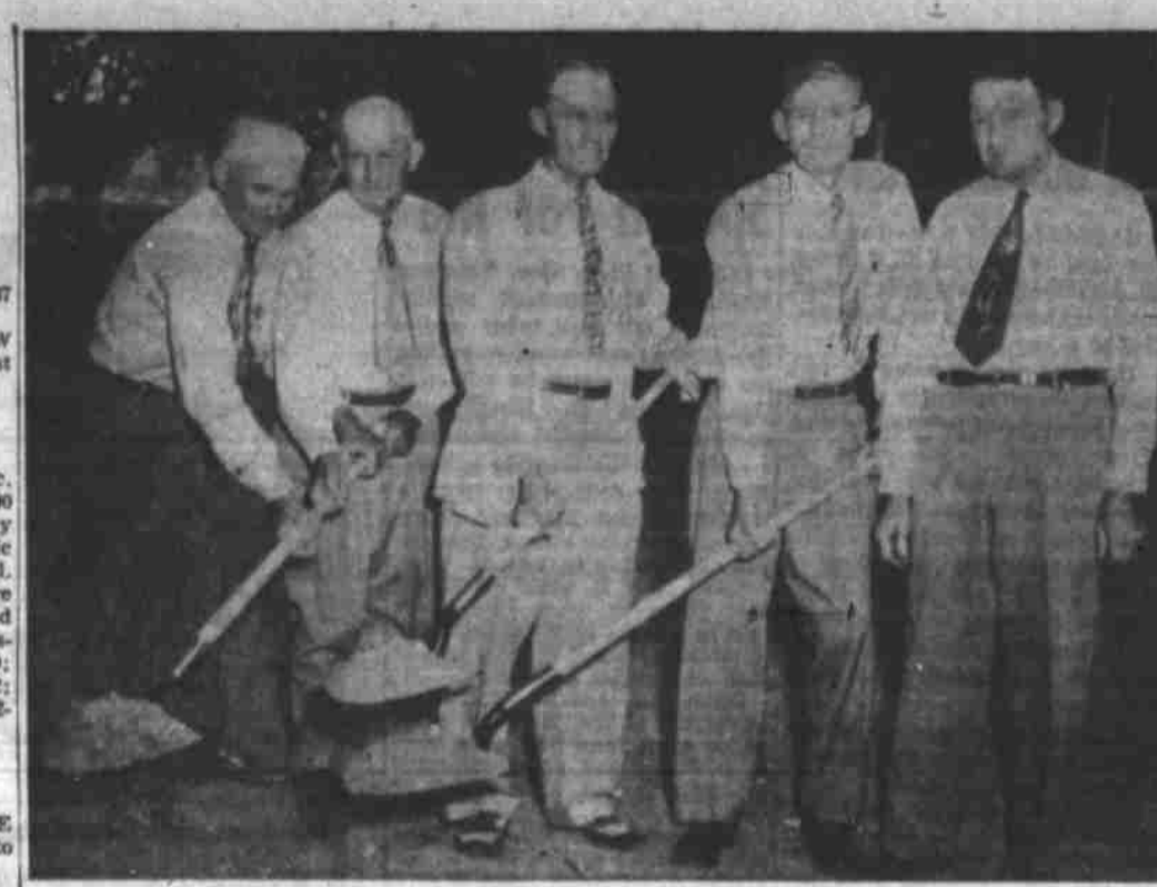
Dirt Broken For New Courthouse
