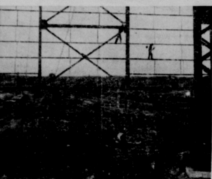
NEW STEEL FACILITIES TAKE SHAPE—Workmen painting braces on the end of a new open hearth building. This new plant is part of the National Production Authority's program for the expansion of basic industry. It will play a major part in raising our steel capacity to 120 million innot tons by the beginning of 1954.
