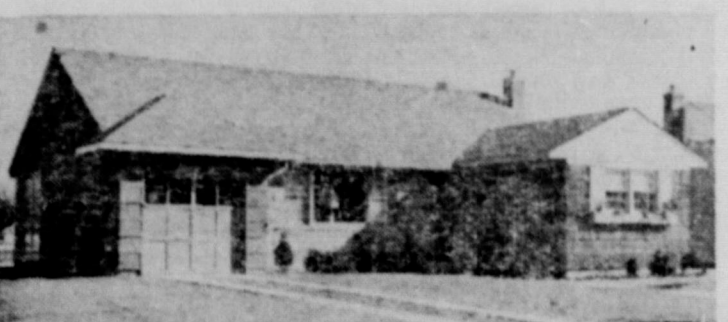
Color scheme for model house above and entire Flower Homes development at Wanliang, Long Island, began with asphalt shingle roofs. Gray-blend is roof color of this house and gray shake shingles are used on the front, sides and rear. Finkish cast of sandstone adjacent to front door gives key to accent color of coral on picture window, front door shutters, scallop on flower box and porch posts at rear. L-shaped kitchen-dinette at left has base and wall cabinets of hardwood veneer which provide attractive, easy to maintain surface.
