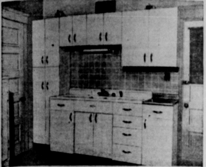
No need to pity the homemaker now. Her modern kitchen saves many hours of hard work. The cost was low because installation of standard steel cabinets and cabinet sink was done quickly without expensive room alterations. Not even the plumbing was changed. Wall tile and a light above the sink are helpful features. There is a lot of work surface on the porcelain enameled top of the steel cabinet sink and on the adjoining base cabinet top. There's lots of storage space made, too. Dishes are washed in the sink bowl and the dishpan has been consigned to the trash pile.
