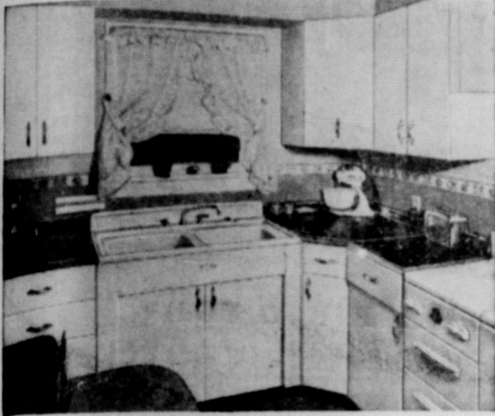
What a change! And the miracle was accomplished in only two days with prefabricated steel kitchen units. Especially interesting is the corner cabinet which uses space formerly wasted. Inside the cabinet are three circular shelves, each 22" in diameter, that rotate with a flick of the finger. The only structural change in the room is the inexpensive wallboard soffit above the wall cabinets. Now the homemaker has convenience galore, with plenty of storage room and counter work surface.
