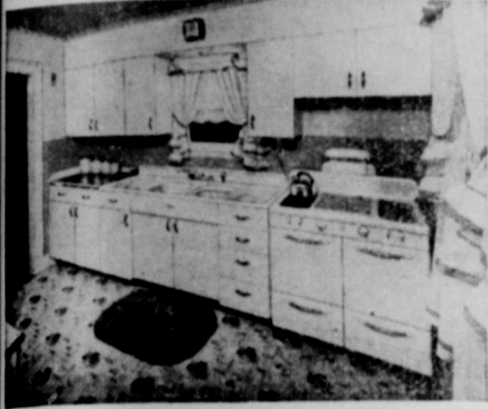
Symbolic of the transformation is the electric clock that replaces the old mantel timepiece. Alterations? Sure, but not expensive ones, because standard steel kitchen units were used and no structural changes were made. The window remains and the new cabinet sink was attached to the old plumbing. A soffit above the wall cabinets and the addition of wall tile are extra features. Note the large number of drawers and compartments in the double-bowl sink and base cabinets.
