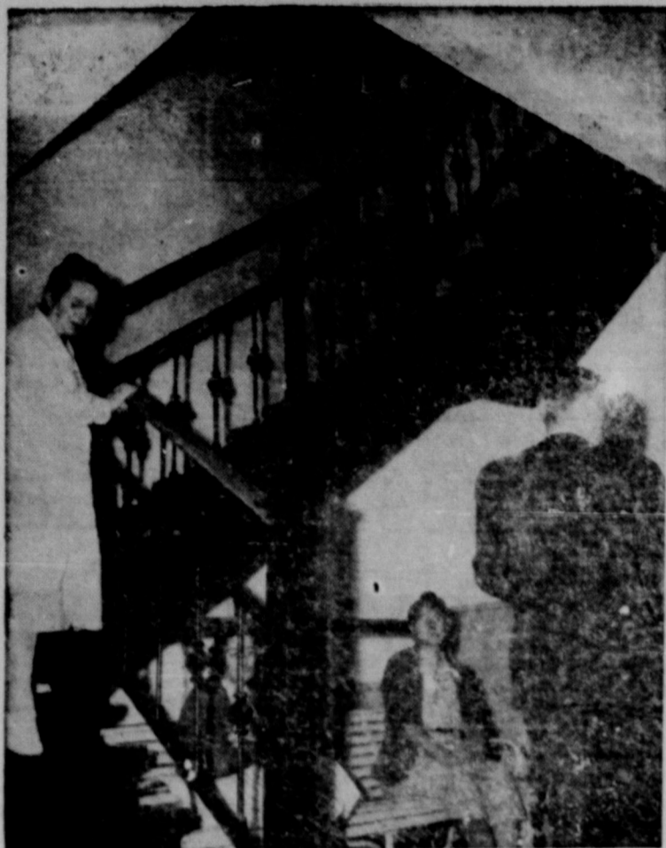
IRON STAIRS IN ABILENE HOSPITAL — This ancient iron stairway at the Abilene State Hospital has caused many falls—not only by the epileptic patients in the hospital, but by the nurses as well. Several patients in the last dozen years have fallen on those stairs and been killed. Injuries occur nearly every week. Notice how cautiously the nurse in the picture is moving from step to step. Abilene State Hospital was one of the several hospitals at which newspapermen of the state recently inspected conditions.
