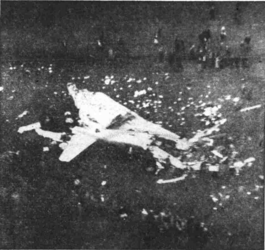
Here is an airview of the spot where the "Sky Chief" transport of Transcontinental & Western airlines crashed to earth near Atlanta, Mo. The terrific impact of the all metal plane is apparent from the wide area over which debris is shown scattered. Note the several clusters of spectators visiting the scene of the air tragedy. (Associated Press Photo)
