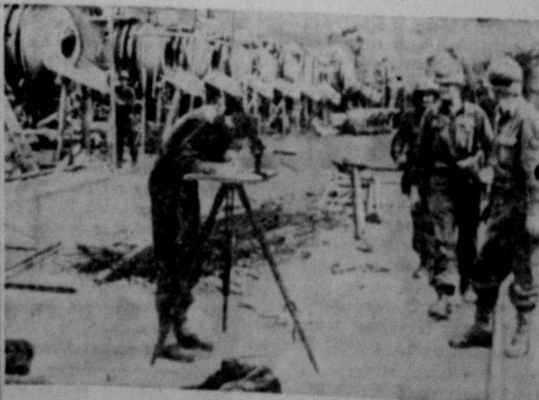
American engineers are shown surveying a 700-foot steel and concrete unfinished ramp in Germany, which is believed to have been planned for use by the Germans as a launching site for rocket bombs. Assembly line of concrete mixers abandoned by the Nazis is in the background. Not enough and too late was the story of this Nazi effort.
