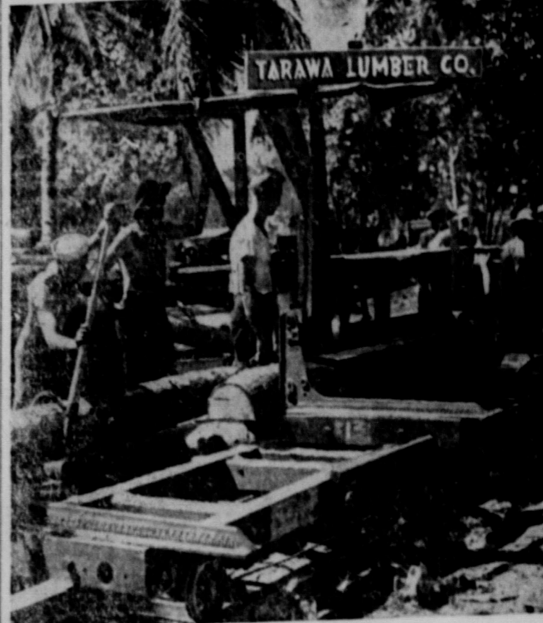
This sawmill was imported to Tarawa to aid in the reconstruction of the former Japanese base after the marines took it in the bloodiest battle of their history. The mill turns out lumber for tent frames, flooring and many other uses. The navy Seabees and marine engineers have done a masterful job in improving this important Gilbert island base.
