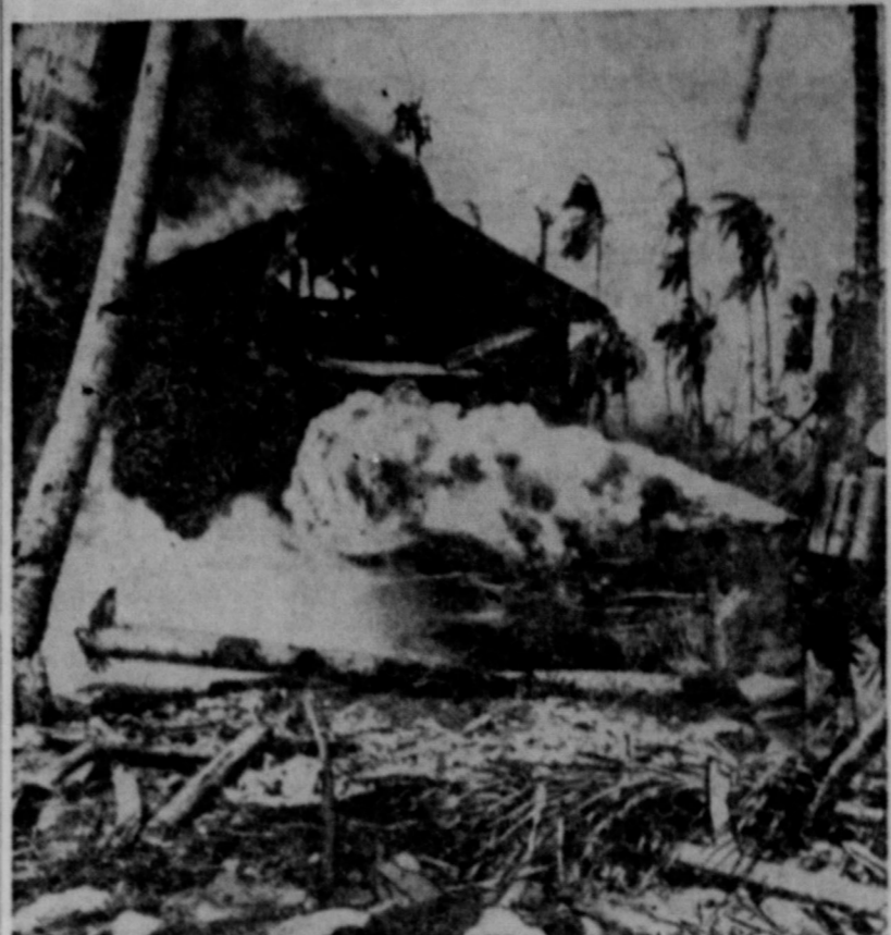
Marine Corp. Elmer R. Burkhalter destroys a partially damaged building on Namur island in the Marshalls with a flame thrower. Roi, Namur and adjacent islands were captured by the Fourth marine division after these areas were subjected to what has been described as the heaviest air and sea bombardment in the history of military operations. In 53 hours 200 tons of bombs fell in this area.
