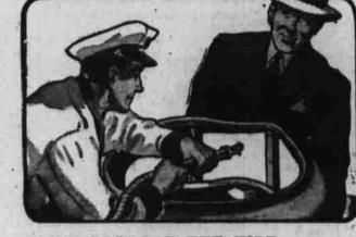
1. WE PREPARE THE TIRE ... First we thoroughly examine the injury inside and out for hidden trouble. Then we ream out the break and cut away any broken cords much like a dentist cleans a tooth for filling.
