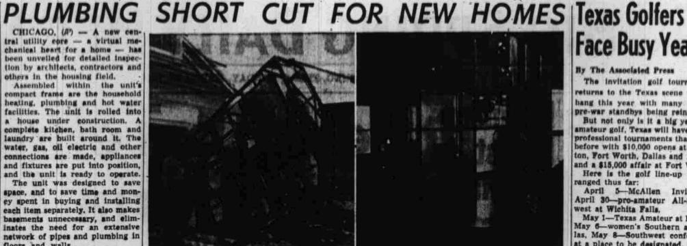
PACKAGED UTILITIES for the new home arrive in one compact unit (left); when installed (right) water, gas, sewer, electrical, heating and ventilating systems of kitchen, laundry and bath connect directly to this core eliminating a network of pipes and conduits under floors.
