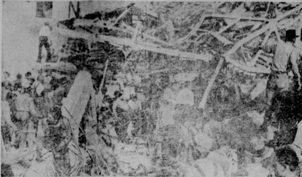
Rescue workers at scene soon after Texas school was blown up, engaged in hazardous task of bringing out the dead.
