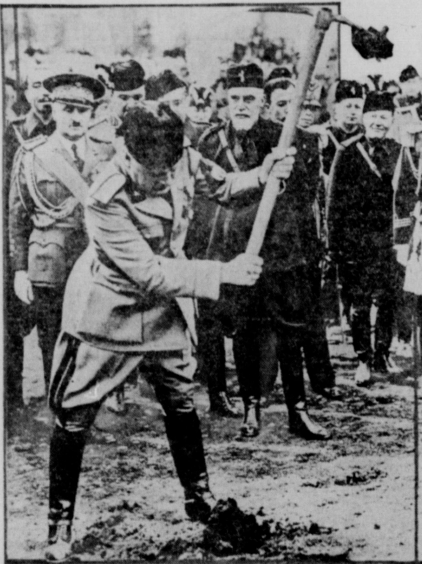
Premier Benito Mussolini of Italy officially starting construction work on the new "Aeronautical City" of Guidonia in the region he has reclaimed from marsh land.
