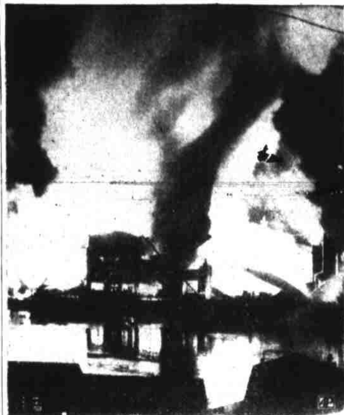
TACOMA PLANT BURNS — Raging flames race through the Western Boat Building and Marine Iron Works plants in Tacoma, Wash. The plants were virtually destroyed. Damage was estimated at more than $50,000. Eleven fire companies and a fire boat fought the stubborn blaze. There were no reports of casualties. Cause was undetermined. (AP Wirephoto)
