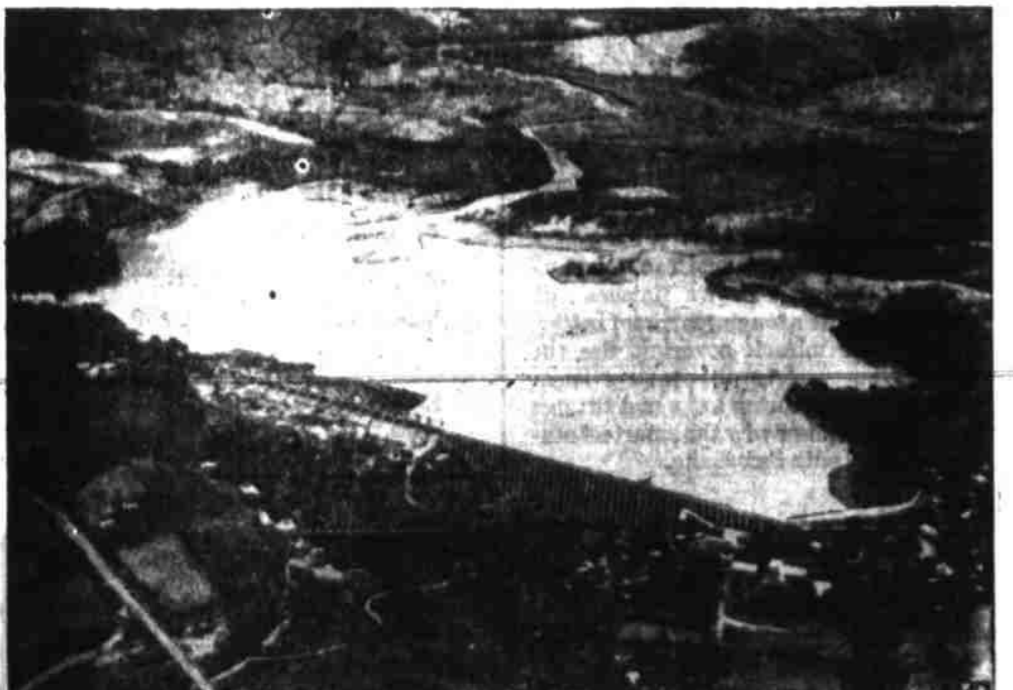
PUERTO RICAN IRRIGATION PROJECT —The Guayabal Dam, on the Yagouas River, impounds water for irrigation along the south coast in the Ponce-Coamo area.
