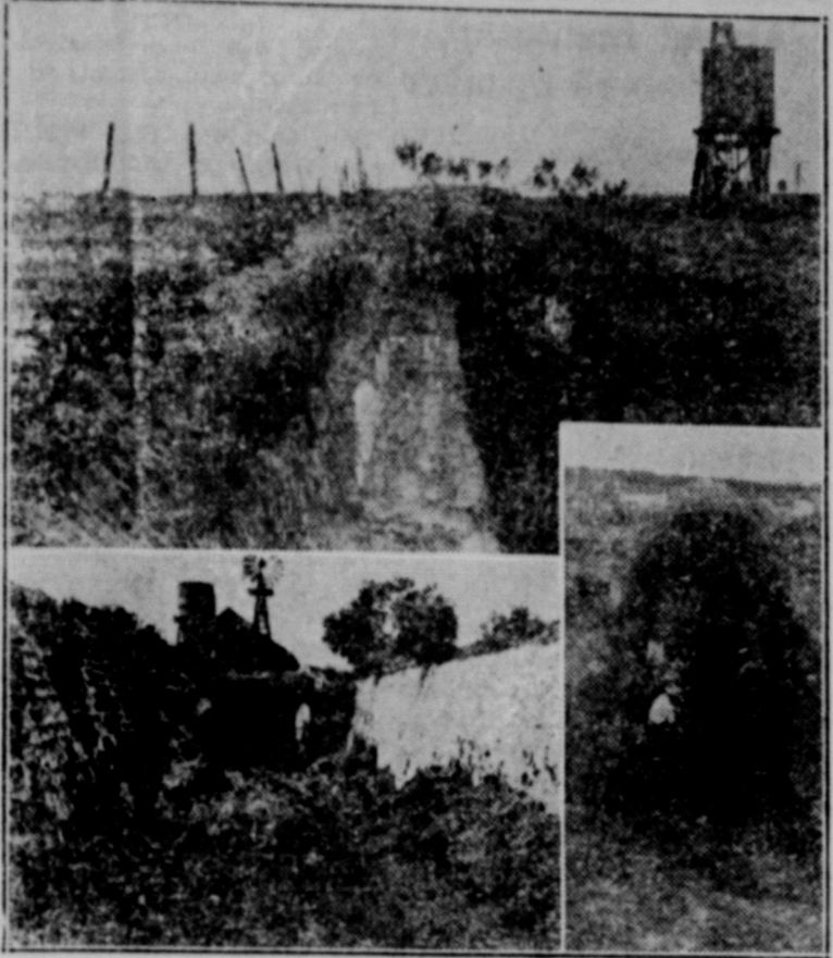
JUST WHAT ITS NAME IMPLIES, a trench silo is simply a trench dug into the ground into which chopped feed crops may be stored for feeding as succulent ensilage to dairy cows, beef cattle and work stock during periods of dry pastures or bad weather. Cheap, easily dug, easily filled, ensilage easily removed, the big disadvantage of a trench silo is excessive spoilage which may be avoided by properly filling, and by providing drainage. More than 200 were dug in Texas in 1931 and county agent reports indicate a big increase for 1932, especially in West Texas.
