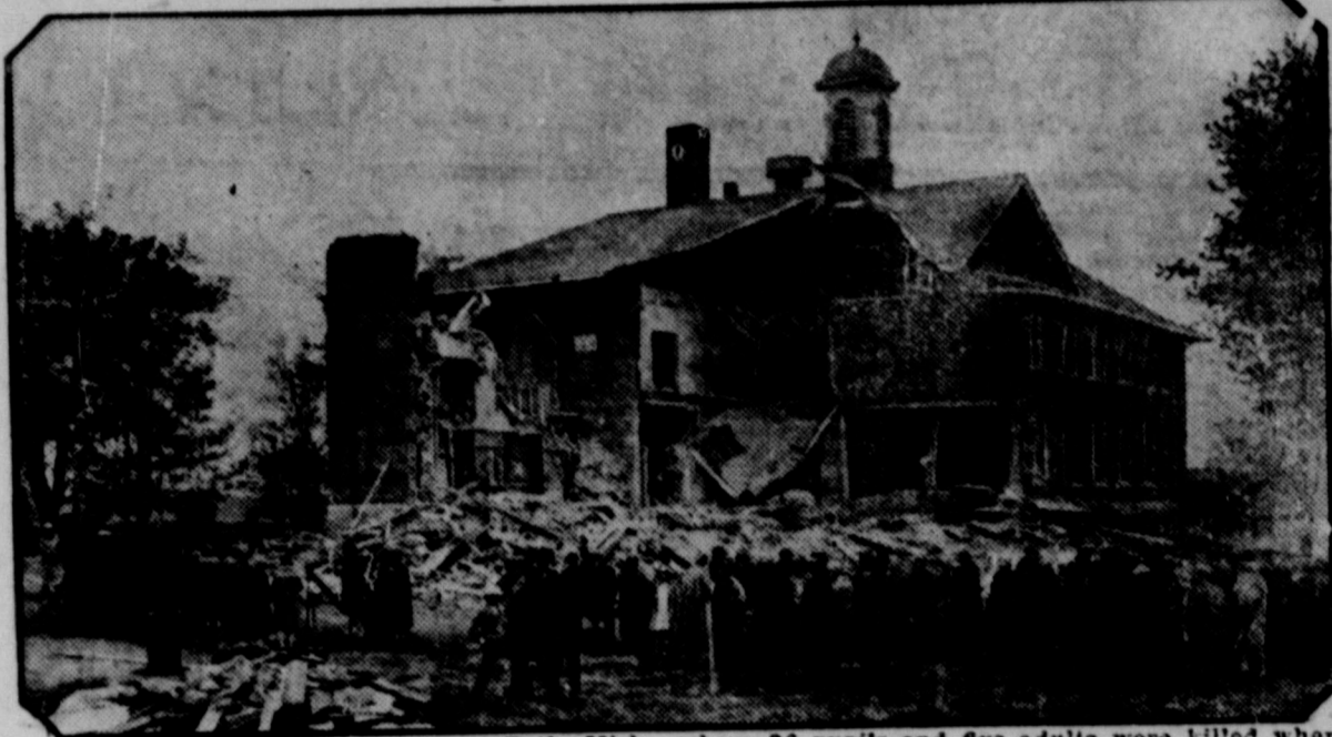
The dynamite-torn schoolhouse at Bath, Mich., where 36 pupils and five adults were killed when the building was dynamited by Andrew Kehoe, demented farmer, is pictured above. Kehoe, believed to have lost his mind when mortgages were foreclosed on his farm, was treasurer of the school board. He met death when dynamite in his car exploded after the detonation wrecked the school.
