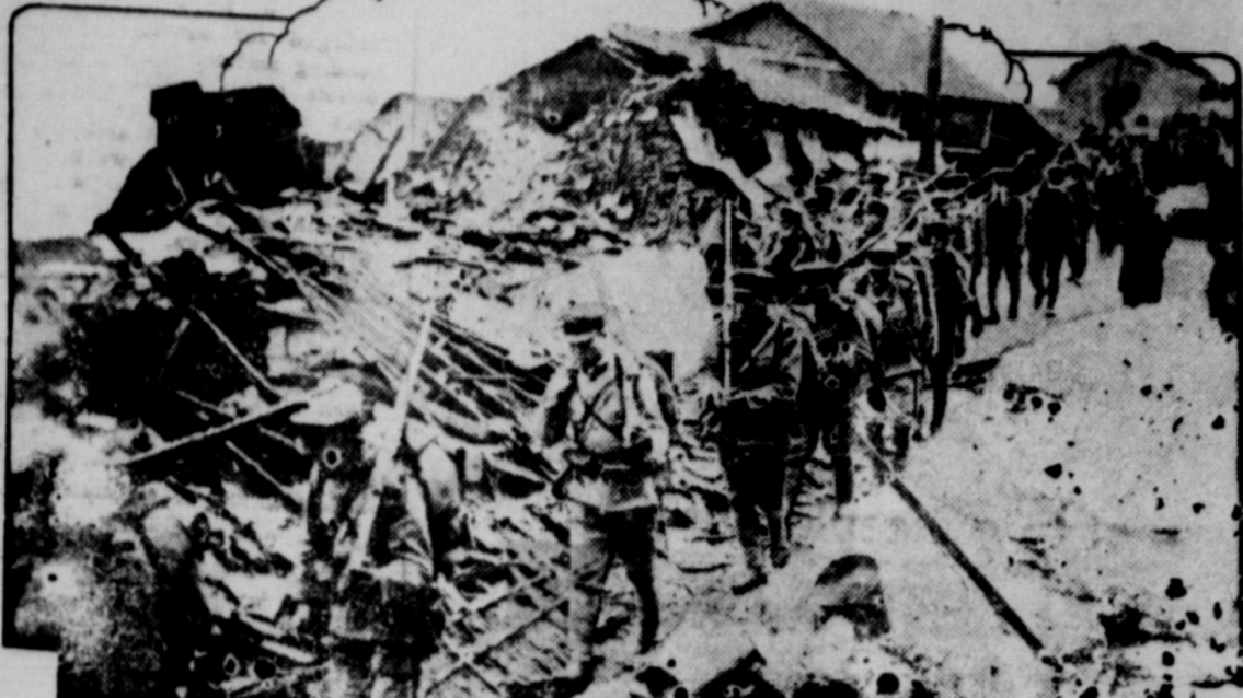
Here is a scene from Mineyama Japan where a recent earthquake claimed 2000 lives. The soldiers are guarding the ruins of stores and homes from looters.
