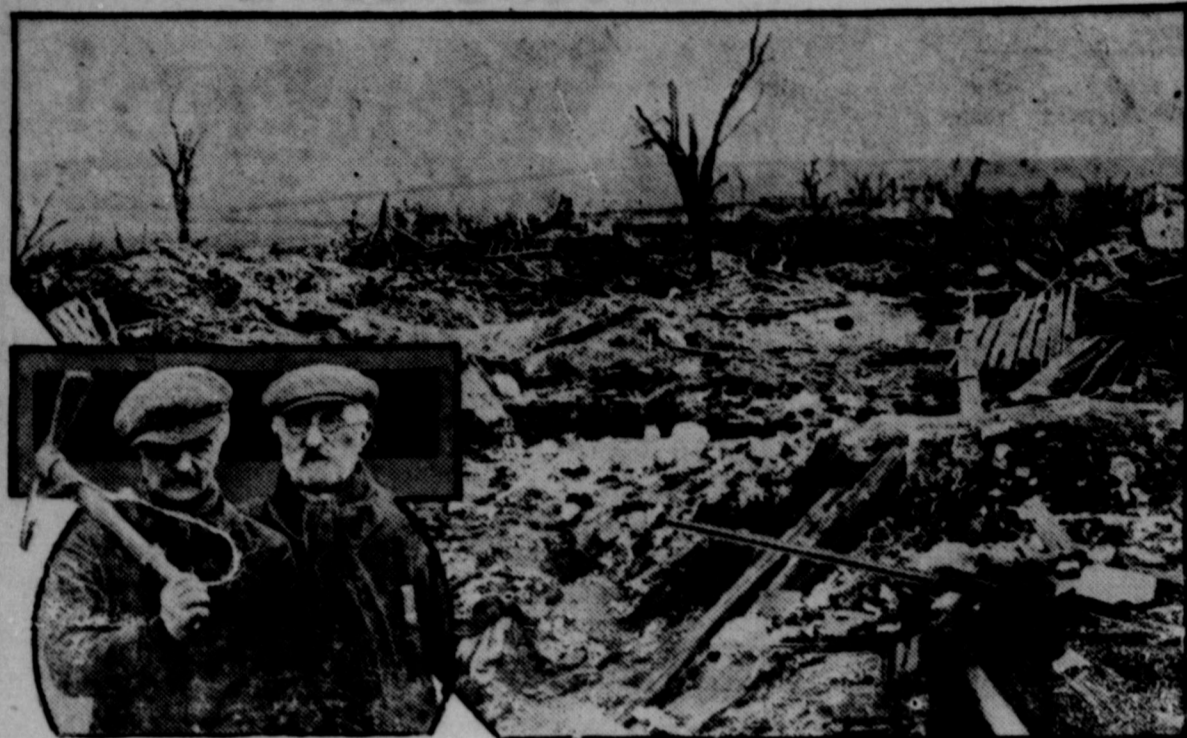
The wreck that was Cantigny June 28, 1918, when American courage under fire was first demonstrated in the World War is pictured above. Inset are Ernest Dubos (left) and Armand Cordier, soldiers who returned from the wars to rebuild their shattered home village.
