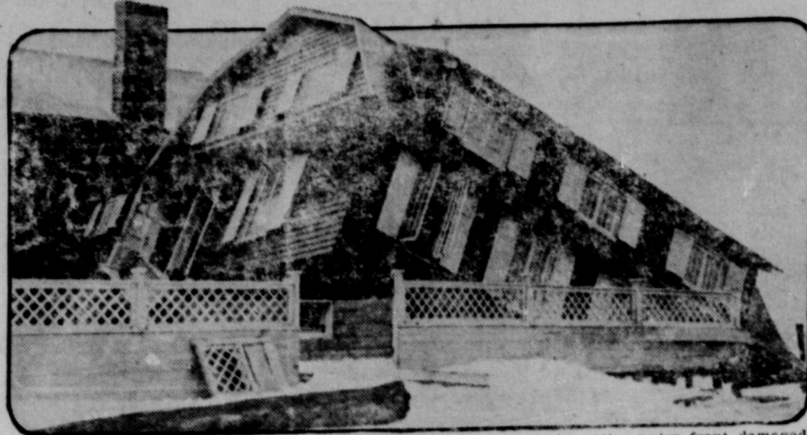
The west end of Long Beach, Long Island, was washed to sea and the entire water front damaged when the worst storm in 20 years lashed the Atlantic seaboard. The house shown above was left topsy-turvy.
