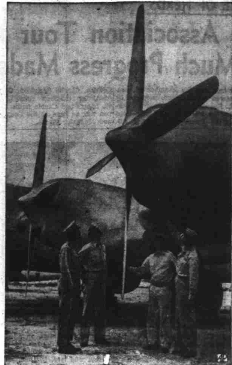
UNDER WRAPS — Officers at the Davis-Monthan Air Base at Tucson, Ariz., check humidity and temperature gauges located behind the glass port on the engine of a B-29 superfortress "cocooned" for preservation. Left to right: Col. N. R. Laughlinhouse, in charge of storage areas at the base, Lt. William C. Anderson, Capt. George E. Scott and Capt. Percy H. Kramer.
