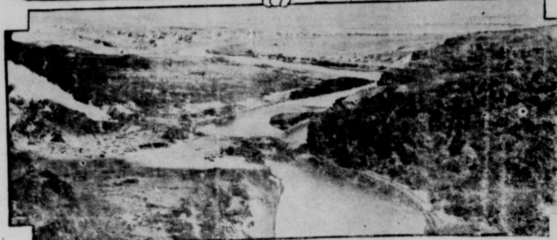
Here is the site of the proposed Boulder Dam at Boulder Canyon, Ariz., on the Colorado river, where 1,000,000 horsepower waits man's bidding. The great natural basin is shown below, where there will be stored 16,000,000 feet of water. The dam itself, to be built at the site shown at the top, will be 550 feet high.
