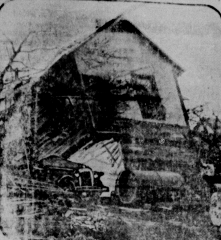
This photo shows a garage-apartment in Miami, Fla., which was raised clear of the foundation by the force of the recent hurricane and left resting on a touring car that had been parked beside it.
