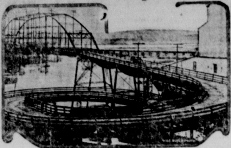
When the bridge across the Mississippi river at Hastings, Minn., was built it was found there was not space for the usual long approach. So the engineers designed a spiral approach, as shown in the photograph.
