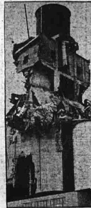
One man was killed and eight others injured at Omaha, Neb., when exploding grain dust and a resulting fire wrecked a tower of the Allied grain mill, which was grinding wheat into feed and flour for the Nebraska-South Dakota drought area. Loss was estimated at $350,000.
