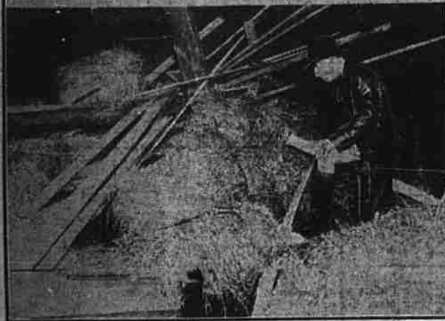
Upper picture shows ruins of a house at Cartersville, Ga., where seven people escaped death by fleeing. Lower photo is of the ruins of a livery stable at Northport, Ala. More than 20 persons were killed in the town of Northport.
