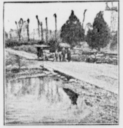
Low Water Concrete Bridge.
