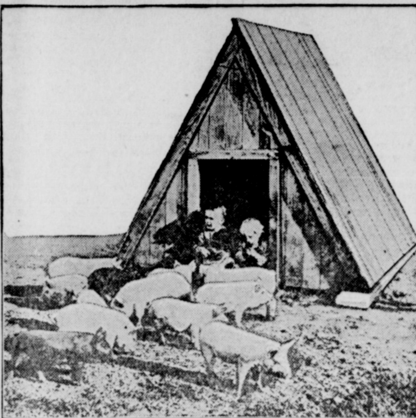
You Can Move the A-Shaped House on Its Runners From Field to Field or From a Dirty Place to a Clean Location.
