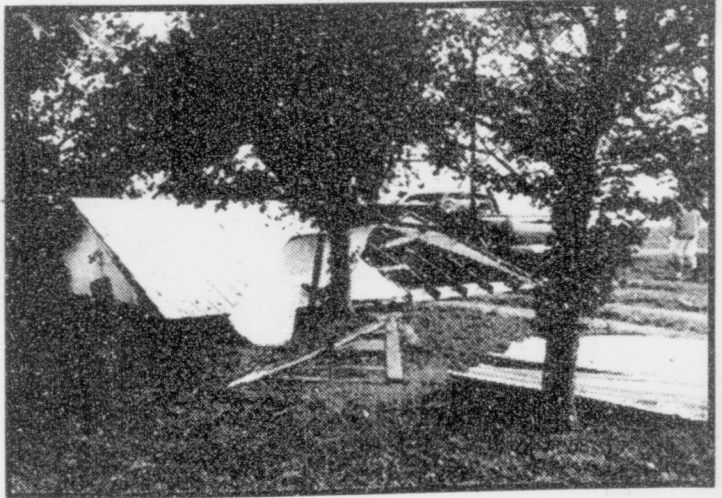
Tony Smitherman's carport was demolished by storms that ripped through the McLean area.
