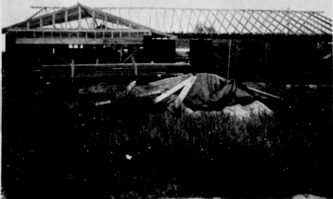
MULESHOE ON THE GROW . . . This example of a new house under construction in Muleshoe shows that Muleshoe is indeed on the grow. There have been many new houses built in the city during the last eight months of this year. Also under construction in Muleshoe are buildings for Muleshoe Motor Company, a new Dairy Queen and workmen are clearing an area for a new bank building for the Muleshoe State Bank. During the past year, Muleshoe has increased in population and also increased in business. Several new businesses have opened here in Muleshoe and of course this week, the Hensley-Russell, Inc. sewing factory will open here.
