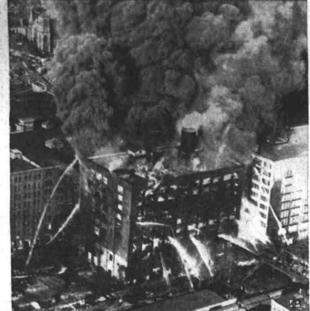
Fire Wrecks Warehouse
