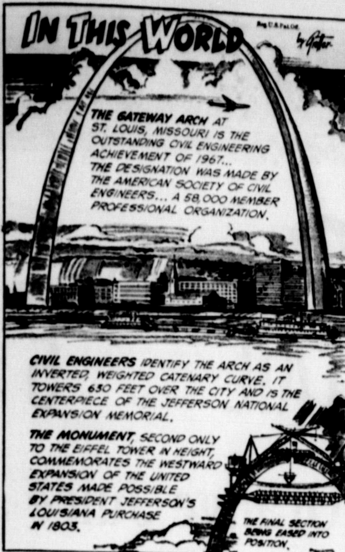
CIVIL ENGINEERS IDENTIFY THE ARCH AS AN INVERTED, WEIGHTED CATENARY CURVE. IT TOWERS 630 FEET OVER THE CITY AND IS THE CENTERPIECE OF THE JEFFERSON NATIONAL EXPANSION MEMORIAL.
