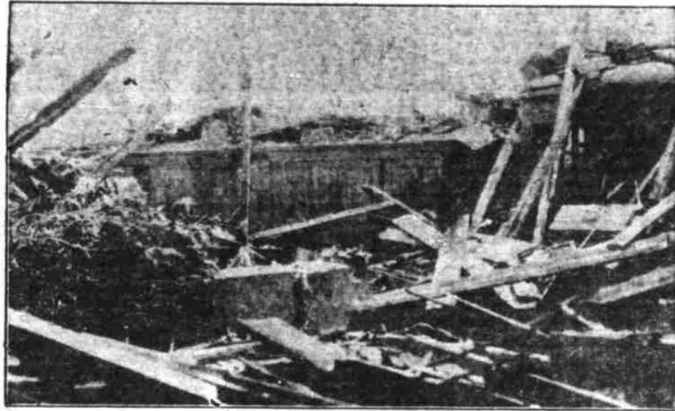
Thirty persons were killed and more than 100 injured and some 2,000 houses wrecked in Gardena, old Cuban town, by a hurricane. This picture shows some of the damage done by the storm and its accompanying 10-foot tidal wave. Damage was unofficially estimated at $5,000,000. (Associated Press Photo)
