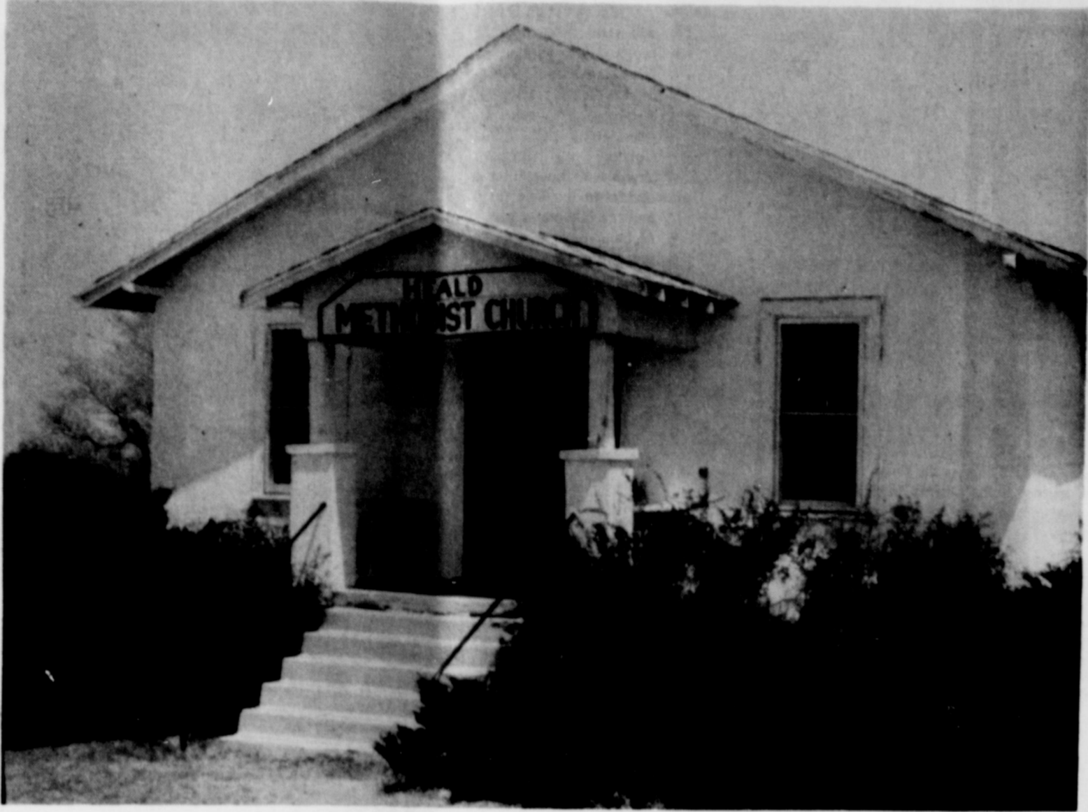
THE HEALD UNITED Methodist Church as it appears today. [Photo by Linda Haynes]
